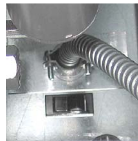
Figure 14 (Rear view of Control Box)
